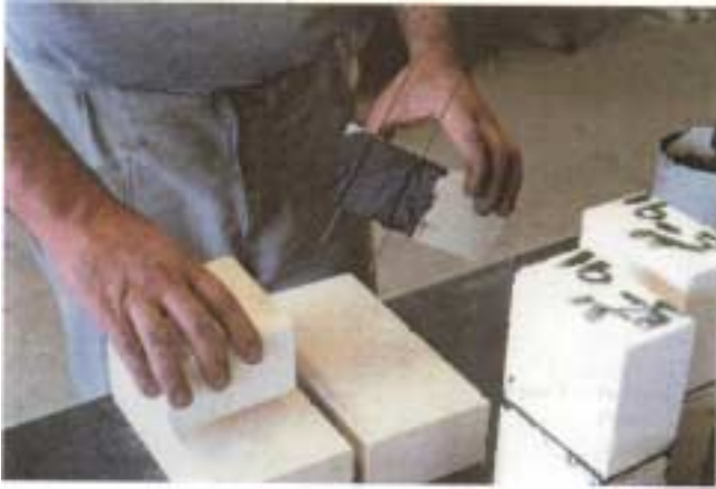
14: I.F.B. 's bonded together either regulated joint thickness (note 2 wires).
